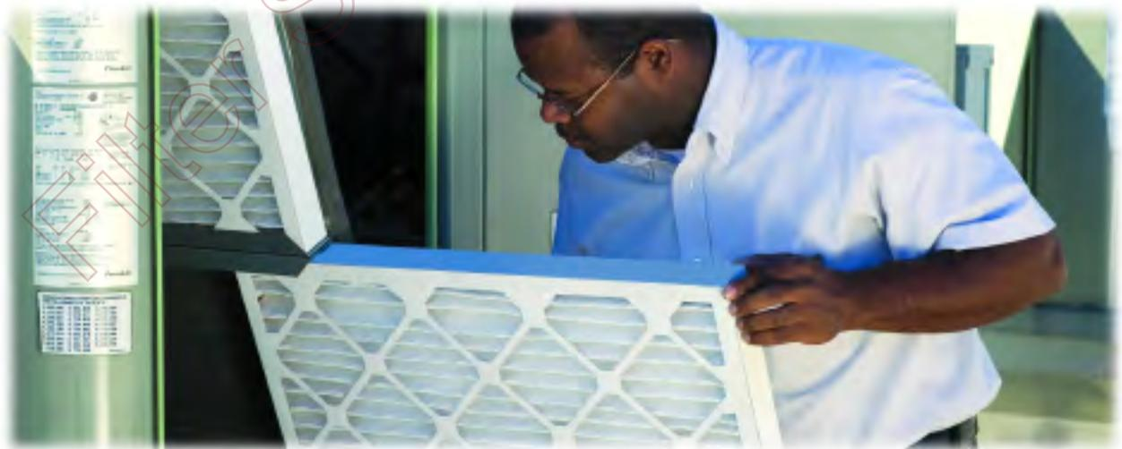
Proper filter maintenance is crucial to keeping HVAC ductwork clean. If dirt accumulates in the ductwork, and if the relative humidity reaches the dewpoint (so that condensation occurs), then bacteria and mold may grow. This is especially the case in HVAC systems with acoustical duct liners, which are frequently used in air handler fan housings and supply ducts to reduce sound transmission and provide thermal insulation.
